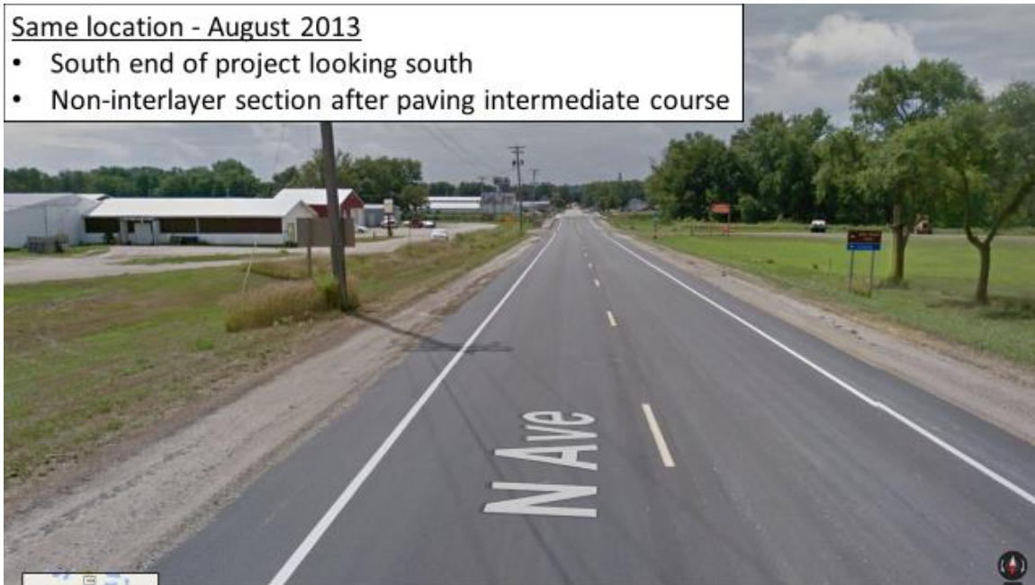
Figure 24. Post-construction view of intermediate course in non-interlayer section on US 169
