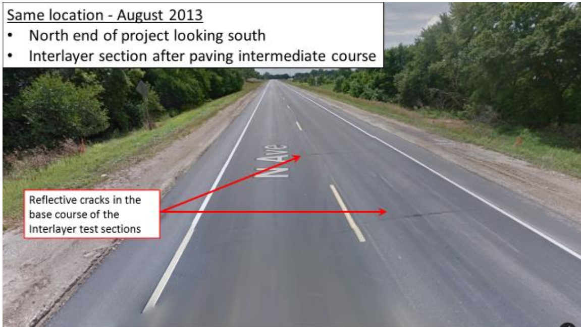
Figure 26. Post-construction view of intermediate course in interlayer section on US 169
