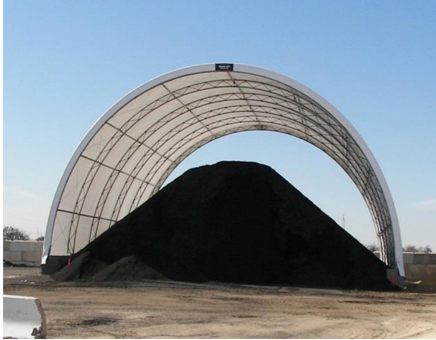
Figure 4. Covered RAS stockpile
