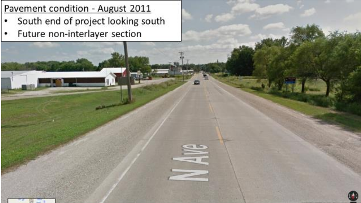
Figure 23. Pre-construction view of non-interlayer section on US 169
