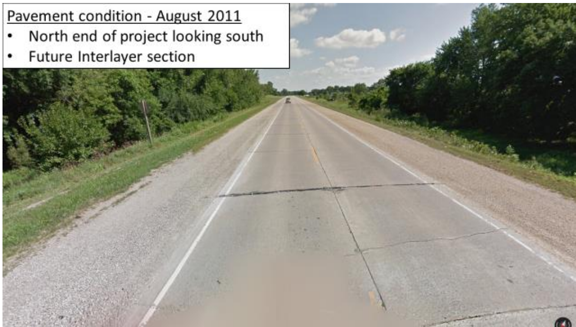
Figure 25. Pre-construction view of interlayer overlay section on US 169
