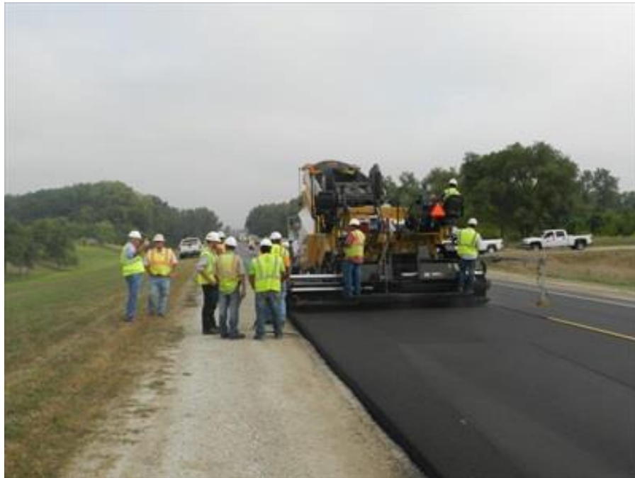
Figure 20. Interlayer paving on US 169
